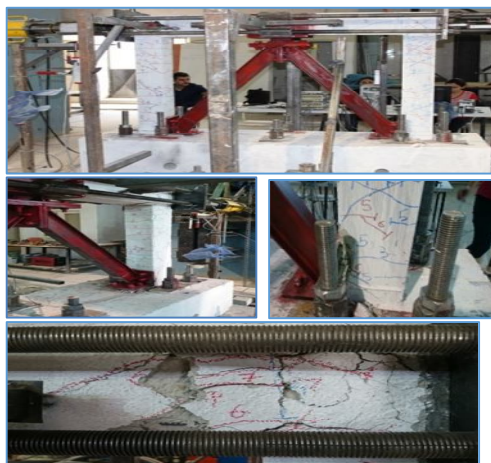
Fig.8. View of the damage occurred after the experiment at retrofitted sample
