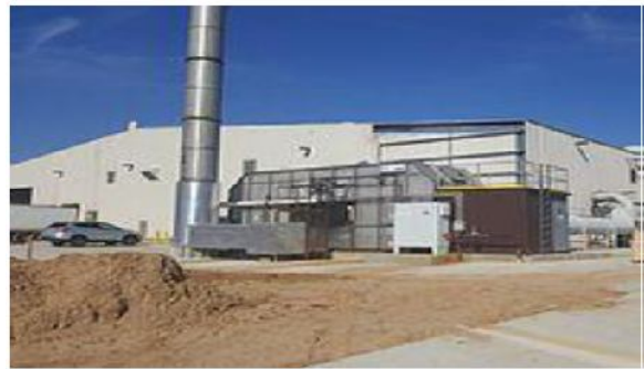
Fig.7 Air pollution control system, known as a Thermal oxidizer, decomposes hazard gases from industrial air streams at a factory in the United States of America
