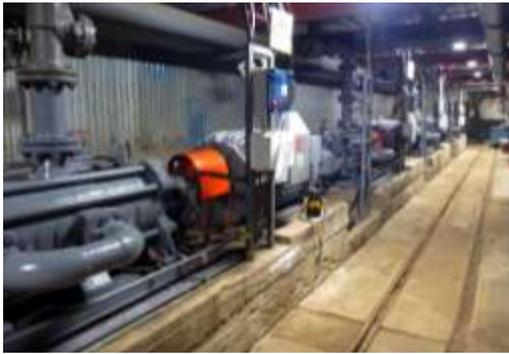
Figure 4: Main pumping station at level 18 in the R3 shaft
