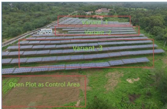
Fig. 5. An aerial view of 1 MW AgriPV plant located at Amrol, Anand
